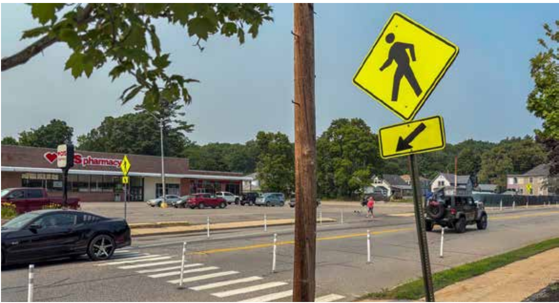
The flexible roadway delineators are meant to narrow the travel lanes and improve pedestrian visibility on the crosswalks. COURTESY PHOTO
