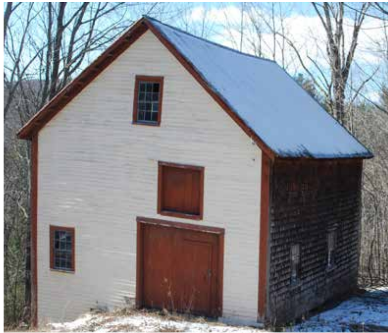
The old apple shed on the former Towle property, now owned by the Newfield Historical Society. PHOTO BY C.J. PIKE
