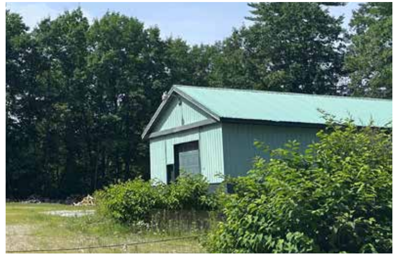
The old Maine Department of Transportation salt shed on Burnham road was the first reported TCE/PCE water contamination site in Limerick for a current DEP investigation. Uncovering the toxic industrial chemicals kicked off several years of investigation into a former Limerick landfill located a few miles away from the shed in an area off Central Avenue near Pleasant Hill Road.
