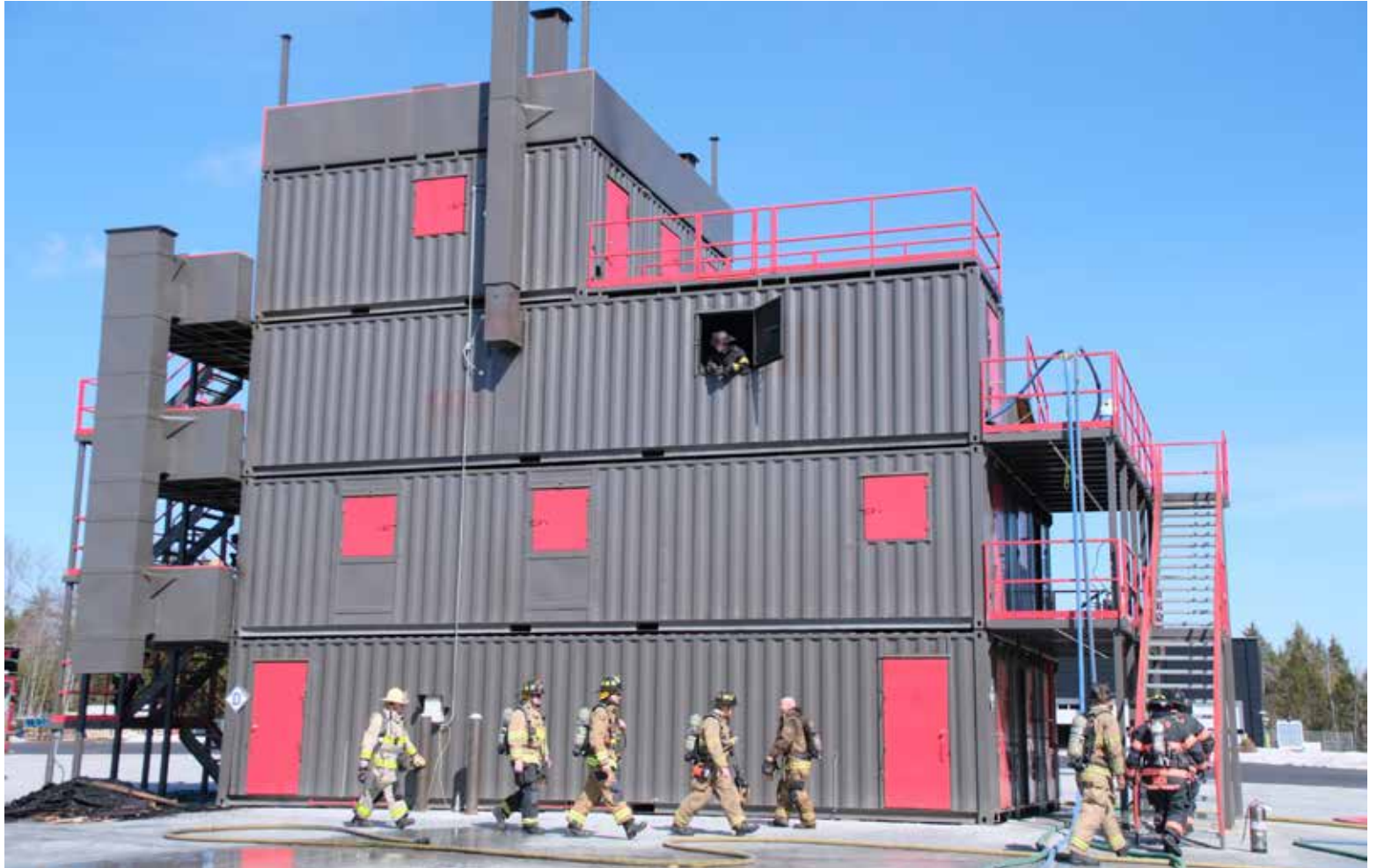
Fire instructors prepare to enter the drill tower on the grounds of York County Regional Training Center in Alfred on a recent day to train on use of the facility so they can train others. The drill tower, made of recycled shipping containers, is also a training tool for law enforcement, EMS, and other first responders. PHOTO BY TAMMY WELLS, YORK COUNTY GOVERNMENT MEDIA
