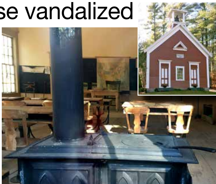
Inside of Washington Schoolhouse, at left is vandalized window temporarily repaired with plexiglass. PHOTOS BY JOANNE BARGIONI
