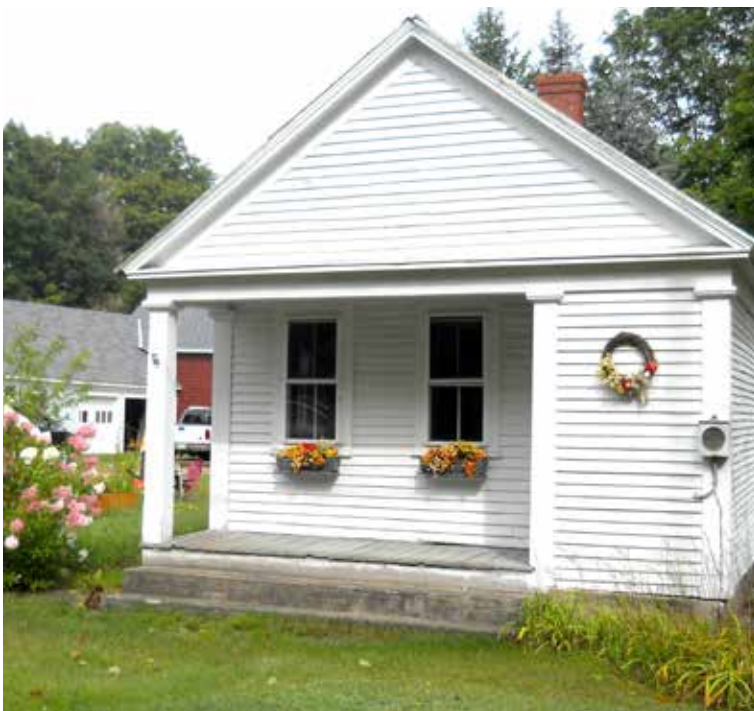
The little building on Elm Street is more than 100 years old, and has been used by lawyers, businessmen and as the town library. PHOTO BY C.J. PIKE
